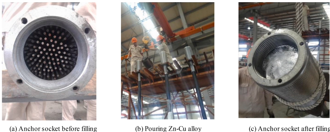
Fig. 2. Construction Process of Filling Media.
